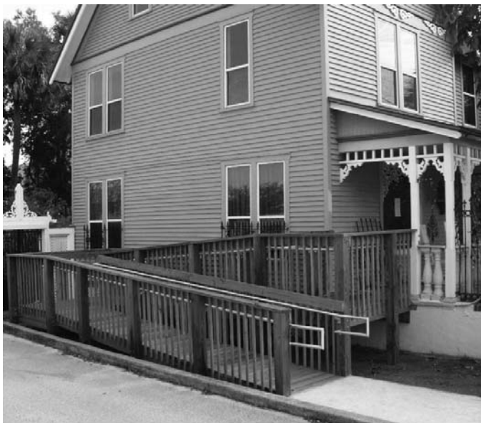
Wooden exterior ramp at the side of a house
